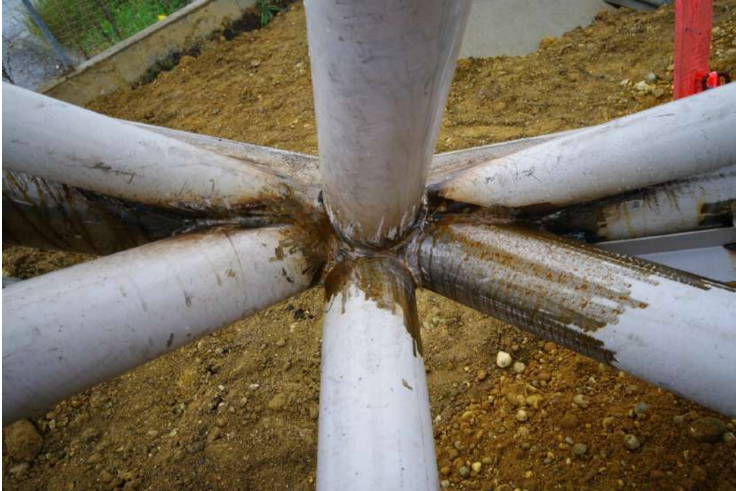
Steel knots without screws
