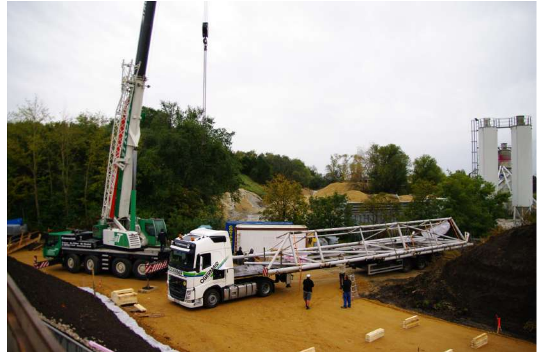
The buildingplot was prepared for assemble the construction
